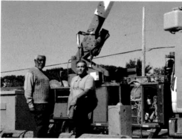
Councilmen Robert Swindle (l.) and James Lauro visit NJDOT road construction site on Rte. 35 and Cliffwood Ave.
