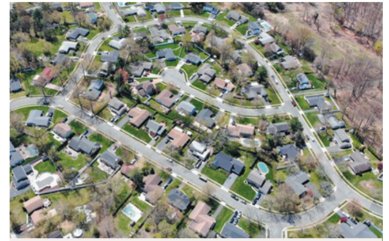
In the Strathmore area's 'D Section,' road reconstruction projects scheduled for next year include Donna Place, plus the portion of Deerfield Lane stretching between both ends of Drexel Lane. This represents the 3rd phase of a multi-year project to fully rebuild Deerfield — the section's longest road.
